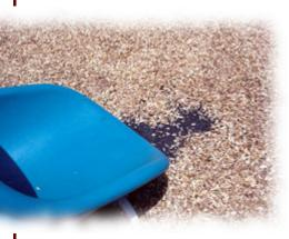
Sof'Fall Engineered Wood Fiber with 6" of Sof'Fall on top. The Sof'Mat should be placed with the Sof'Fall Engineered Wood Fiber surfacing mounded in the middle of the mat. The corners of the Sof'Mat should be tucked into the Sof'Fall Engineered Wood Fiber to help
